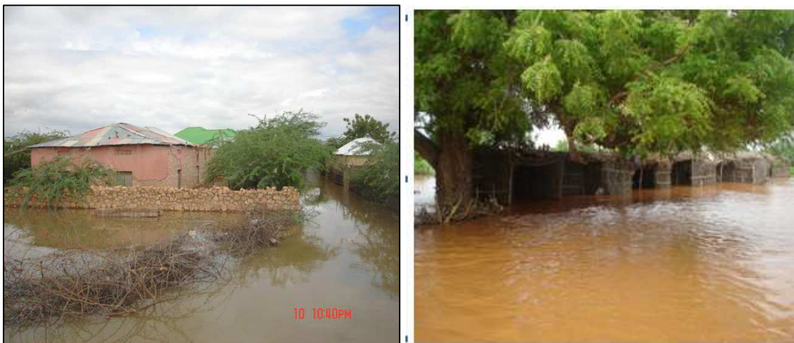
Figure 12: Pictures of flooded houses in different areas in Somalia in 2006 floods
