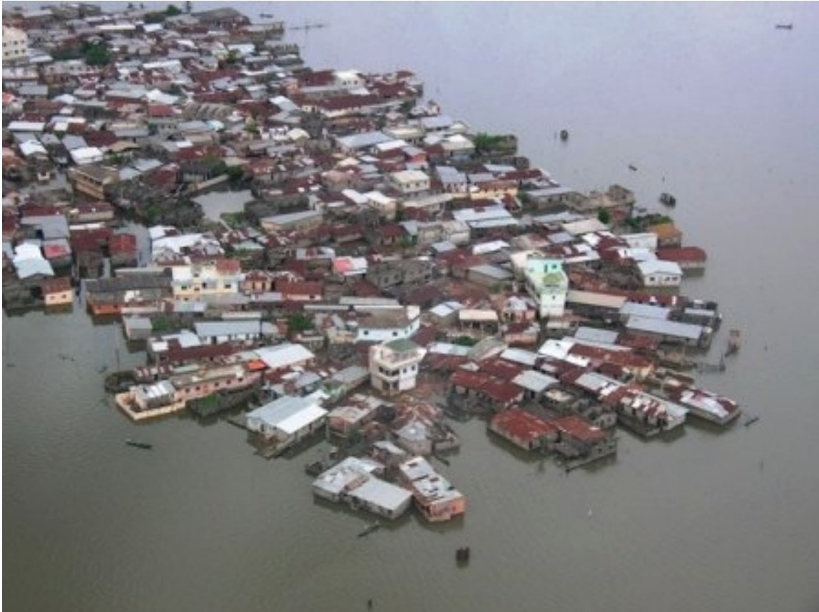
Figure 12: Neighborhood in Benin caught by the rising waters during the recent floods
