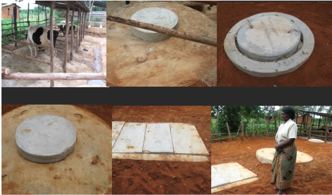
Figure 21: Biogas Digester Project
